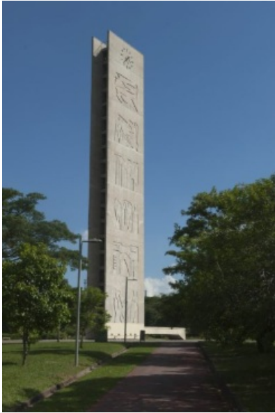
View of the Clock Tower on the Butantã campus of the University of São Paulo. Photo: Julio Bazanini
